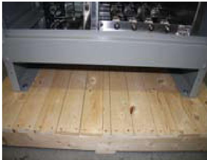
PHOTO #10: 11/16" holes provided at each enclosure frame leg
