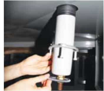
Photo #7: Bushing Assembly Step 4
